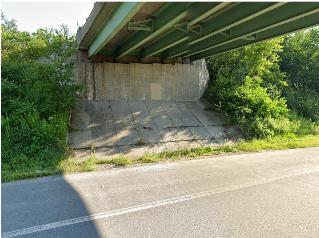
Photograph 3 – Abutment No. 2 (south side of existing bridge) supported on steel HP14x73 piles.
