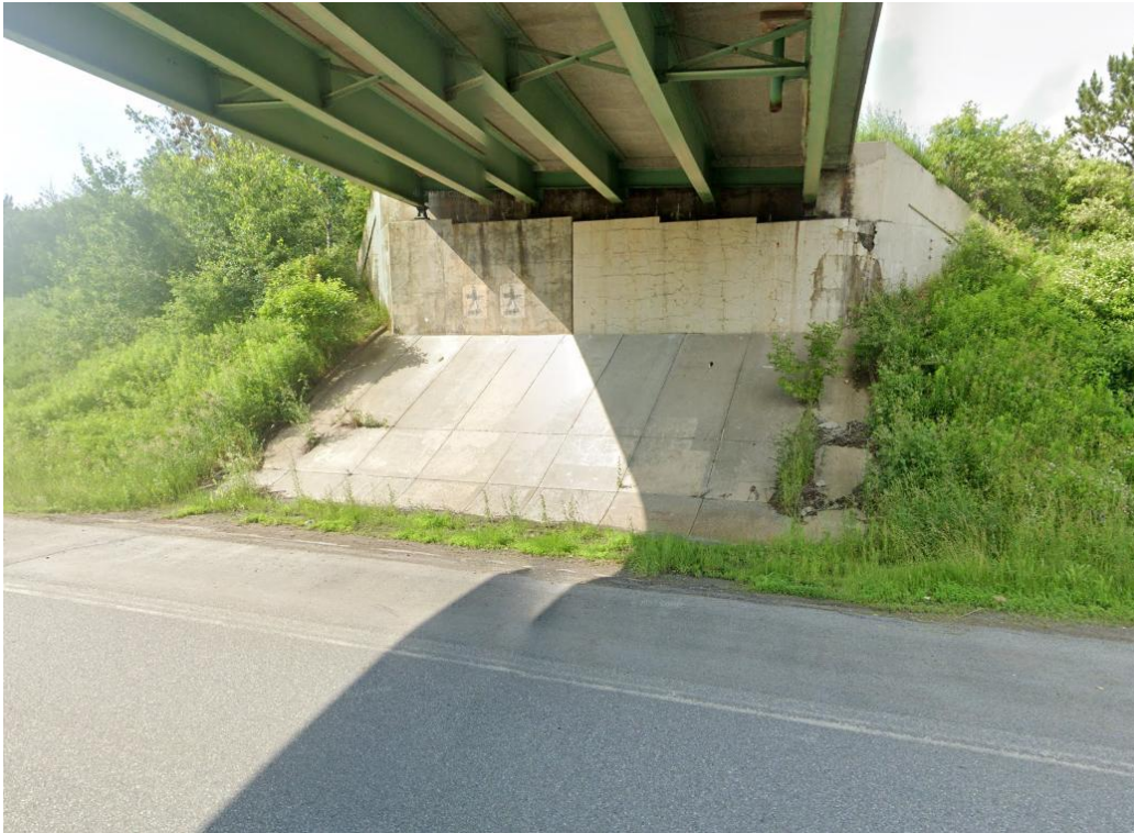
Photograph 1 – Abutment No. 1 (north side of existing bridge) supported on steel HP14x73 H-piles.
