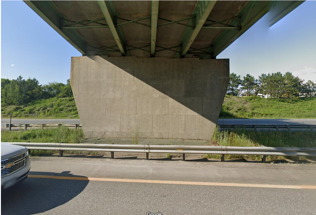
Photograph 2 – Pier supported on steel HP14x89 piles.
